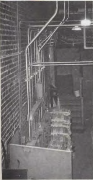
The basement of our school.
